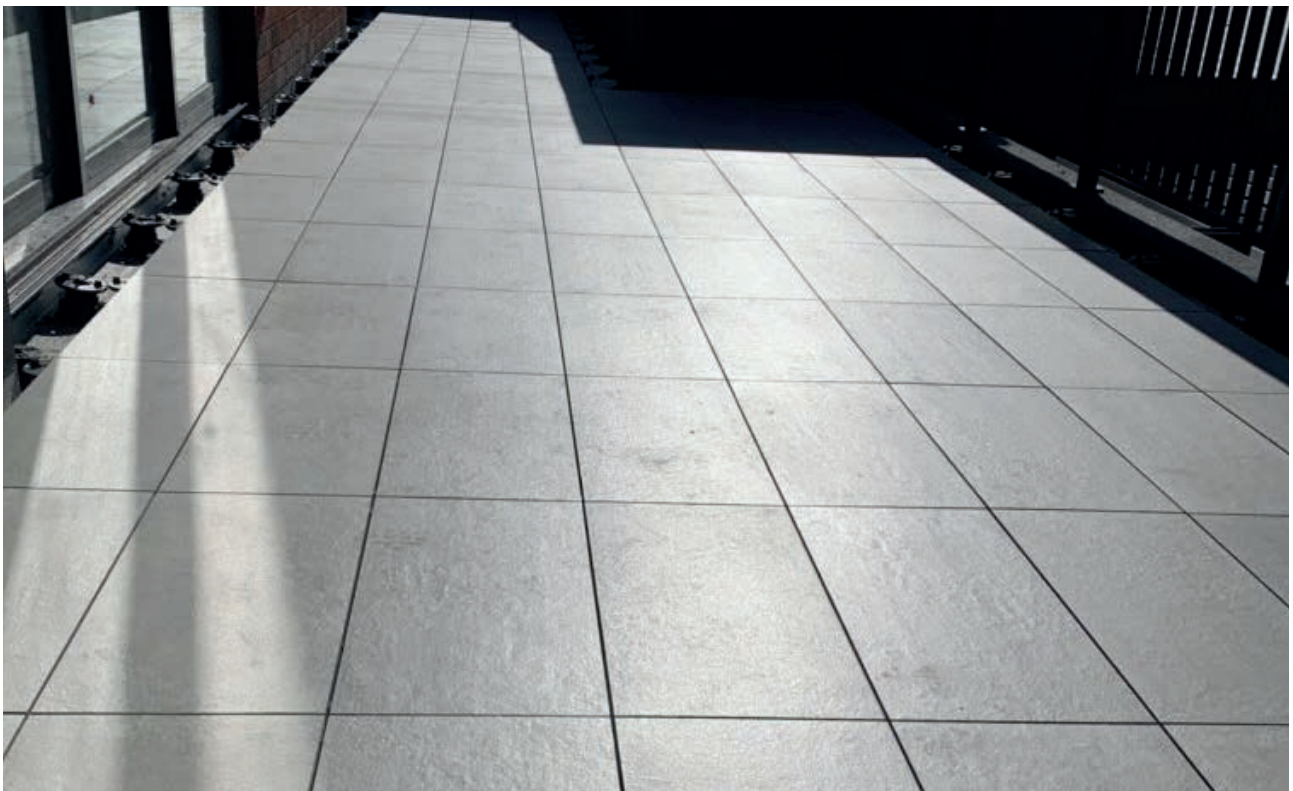
Clifton Crescent Mount Lawley – Rooftop, terrasses et espaces extérieurs Perth, Australia Pedestal System – Basic SB
