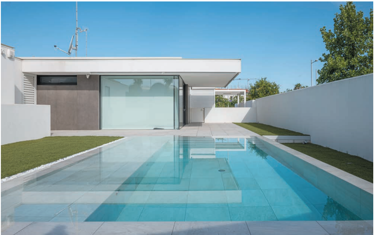
Villa privata – Bord de piscine Jesolo (VE), Italia GRF System – Pedestal Prime®
